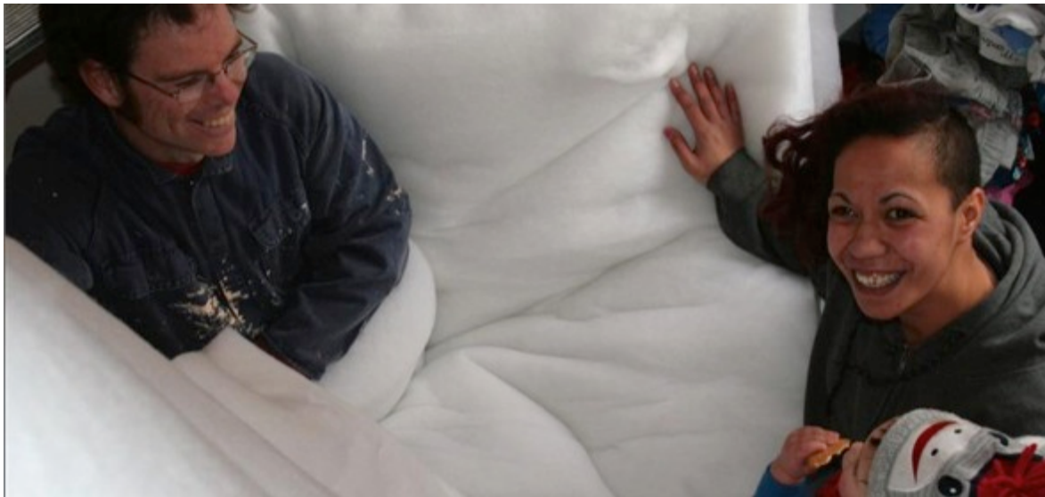
Transition Valley 473 member Alex King and resident Cassandra Thomas, with her nephew Hemi Birch (1) watch the new insulation go up into the ceiling of Ms Thomas' home. Photo by Dan Hutchinson (The Star)
