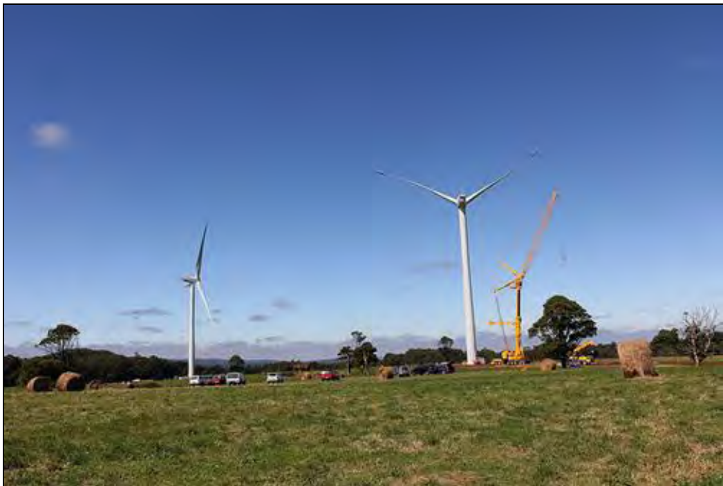
Hepburn Wind Farm during construction, 2011.
